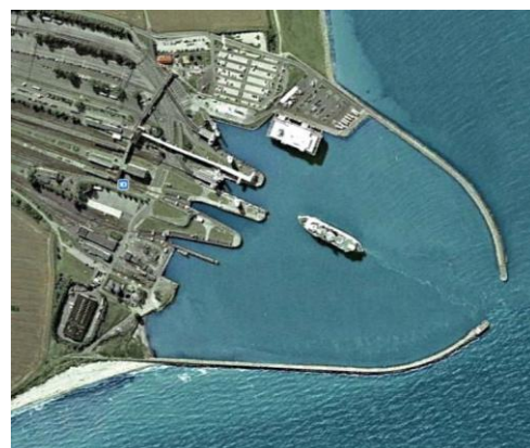
Fig. 2. Aerial view of ferry terminal
