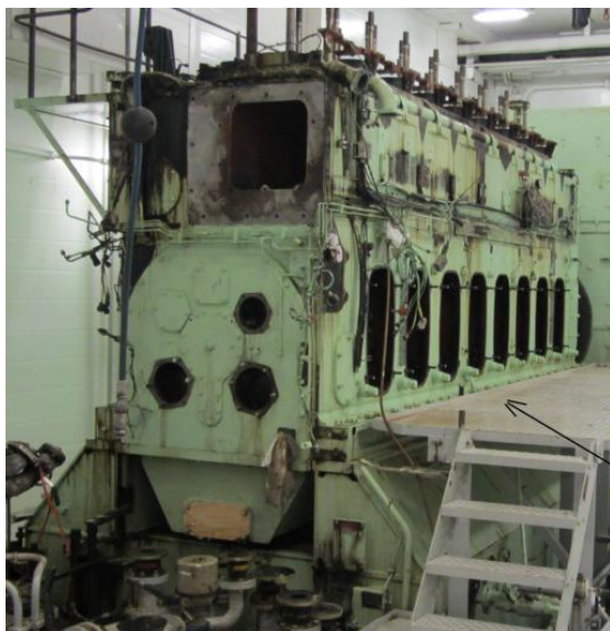
Dismantling of a 3520kW Diesel engine
