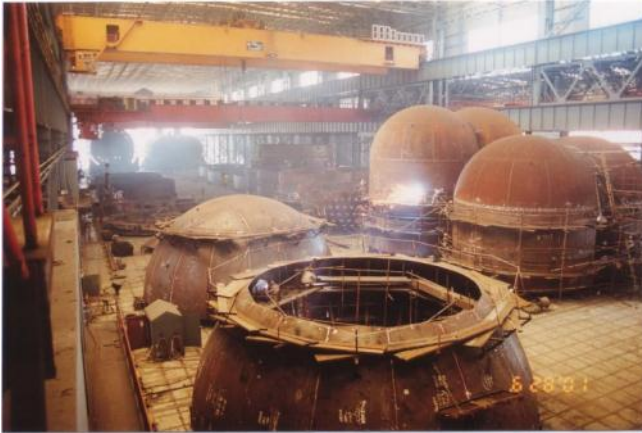
Fabrication 8,200 m 3 and 8,400 m 3 Bilobe and Cylindrical Tanks for Ethylene Service
